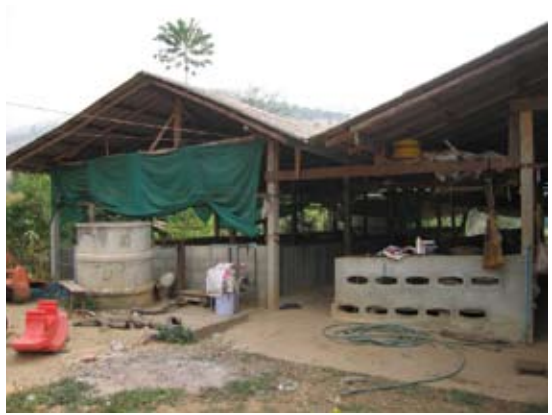
Photo 10. Large concrete pig house (March 2010, village B)
